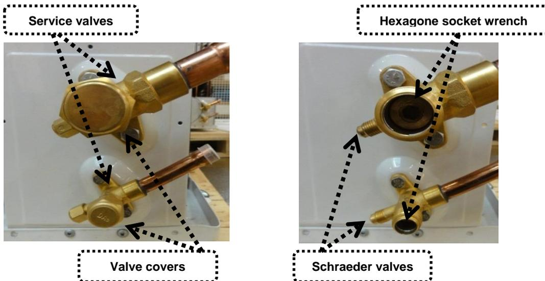
Figure 26: Service valves for refrigerant charging
