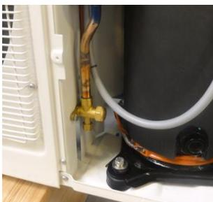
Figure 27: Liquid line service port
